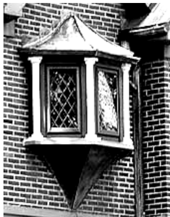
Oriel with small window panes.
